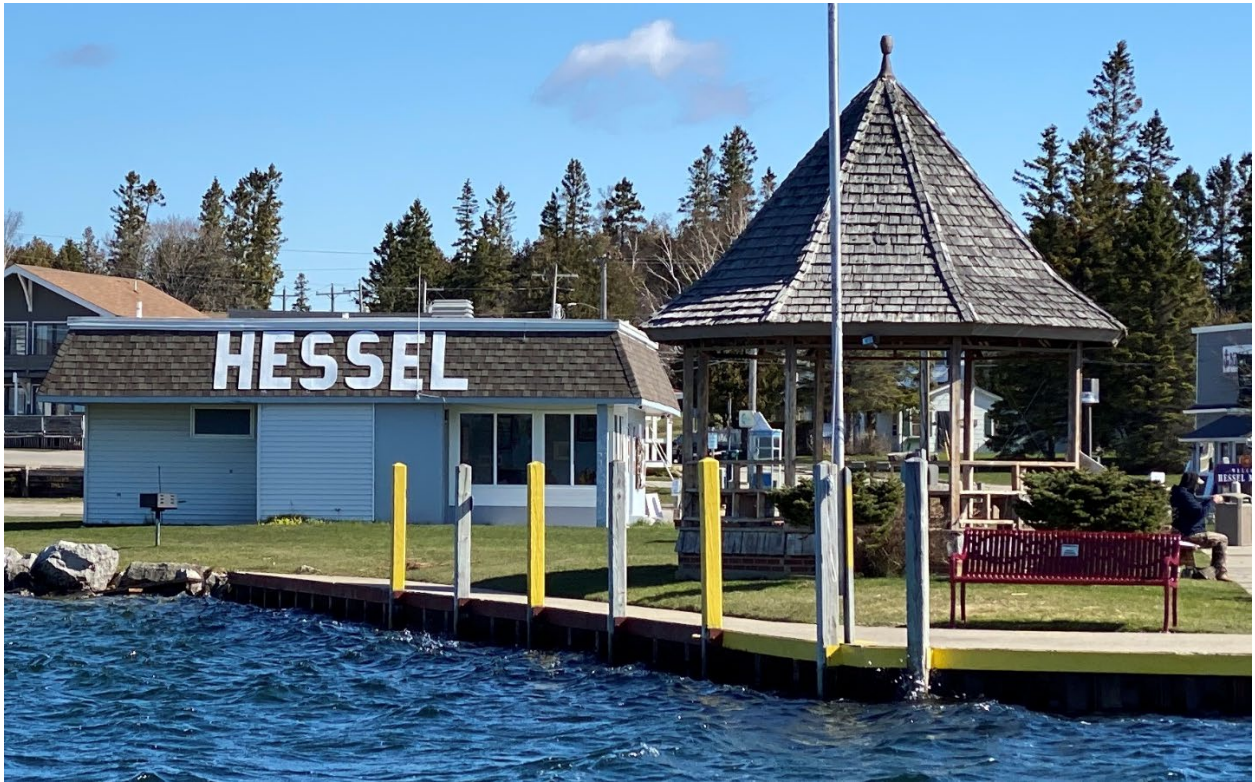
Boater Services Building South Elevation
