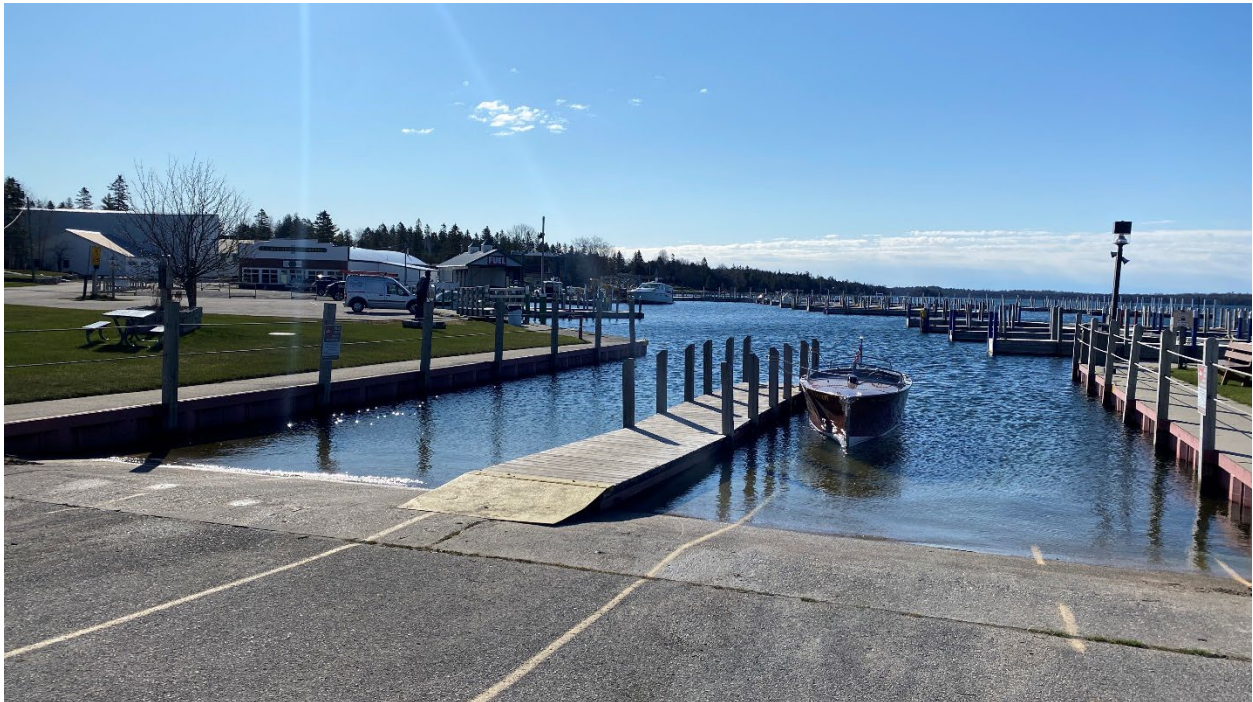
Existing Boat Launch and Perimeter Walks
