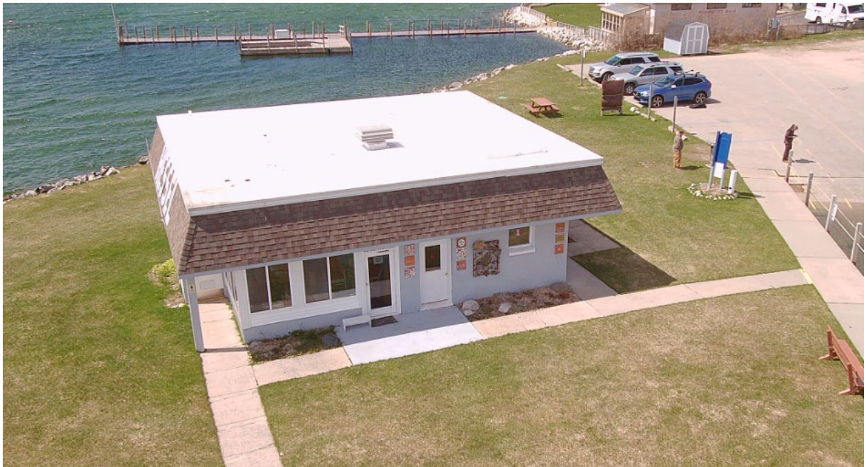
Boater Services Building East Elevation and Roof
